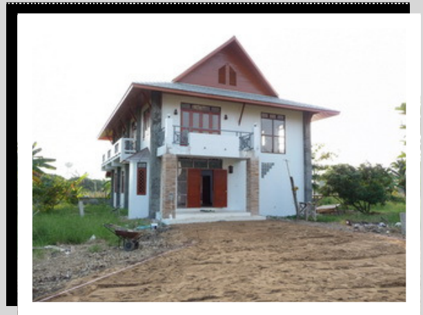
Before the work begun
