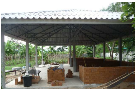
The construction of the organic farming facility.
